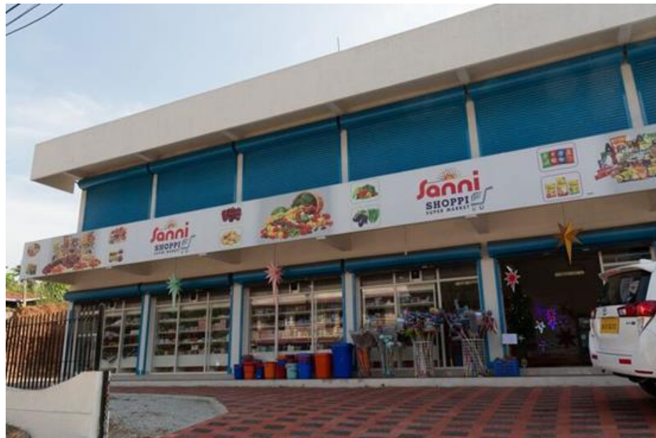
Exterior (the upper floor would be expanded)
